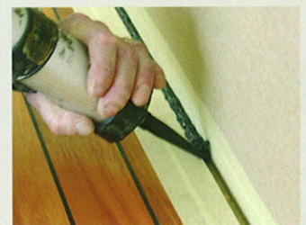
6 – Apply a peripheral joint " NAVYJOINT " and smooth it
