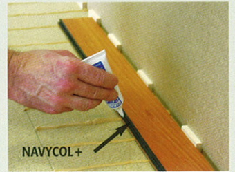
2 – Gluing of tongues with NAVYCOL+
