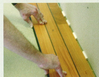
5 – Apply then the blade to its length
