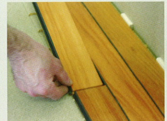
4 – Place the blade on the extremity of the previous one
